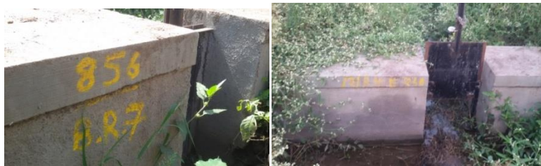
Figure 19: Image of minor gate with chainage and gate number
