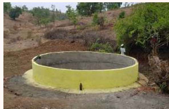
Rejuvenation of drinking water well at Rajewadi, Jawhar Block
